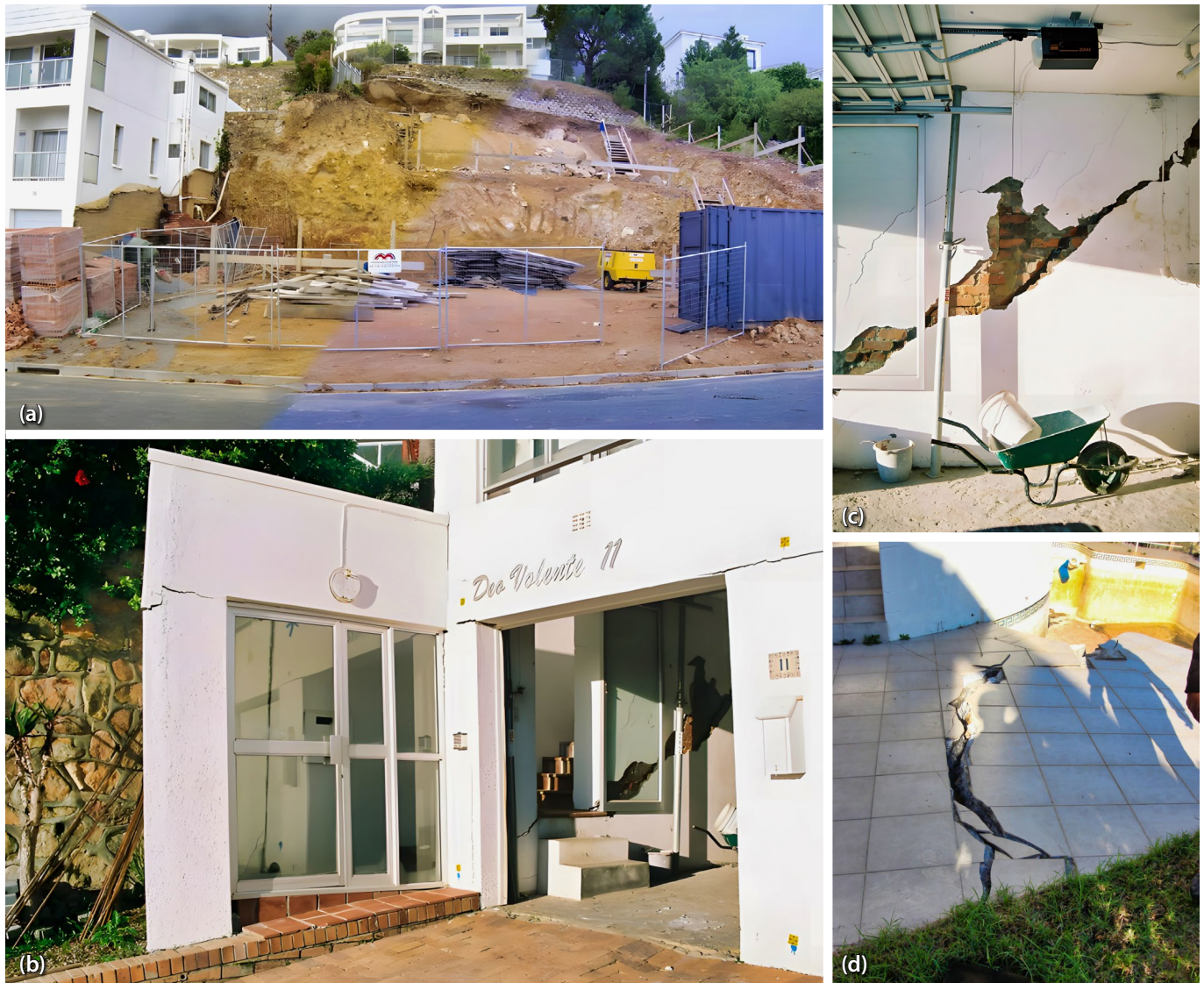
Figure 2 (a) Unsupported cut created in Barbara Road, Camps Bay, (b&c) damage to the adjacent house, and (d) damage to the house above the cut
