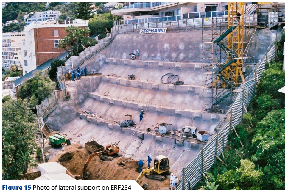
Figure 15 Photo of lateral support on ERF234
