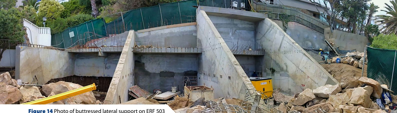
Figure 14 Photo of buttressed lateral support on ERF 503
