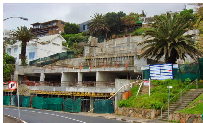
Figure 5 Lateral support at Boulder apartments
