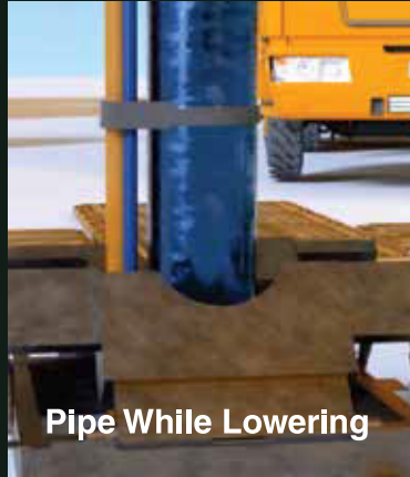
Install the HCL Cable Clamps to the ZSM Riser Pipe while Lowering the Column
