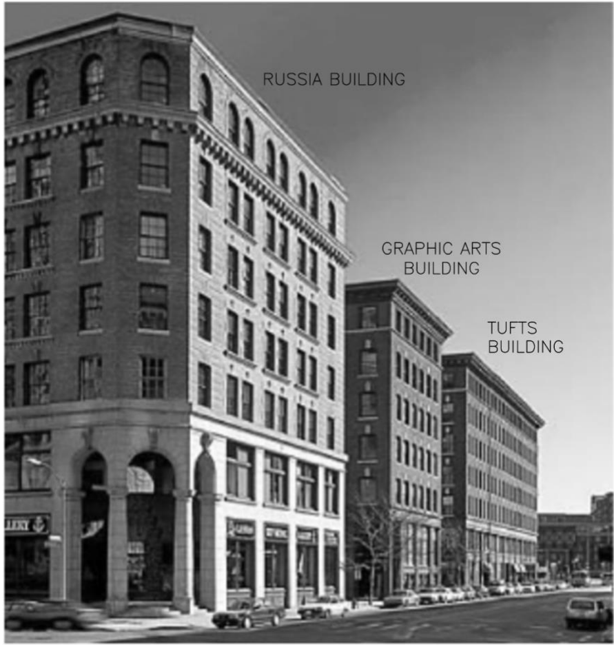
Figure 1. Russia Wharf Buildings, facing east.
