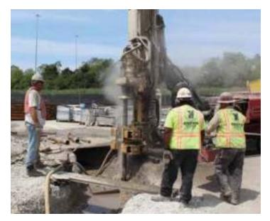
Dewatering removes groundwater from a construction site, usually via pumps. Griffin has a variety of systems, from simple sump pumps to deep wells. The best solution depends on factors that are unique to every site—everything from soil permeability to stratification.
